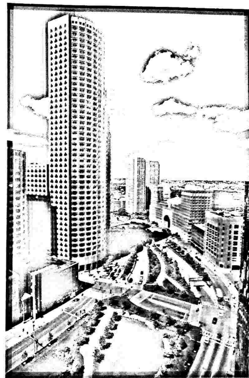
▲ FIGURE 13-55 FREEWAY DEMOLITION Boston's Central Artery freeway was demolished and replaced with the Rose Kennedy Greenway.
